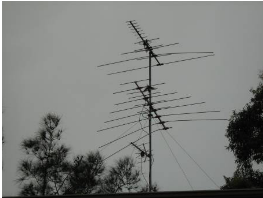
Figure 1: Aerials with damaged or broken elements
